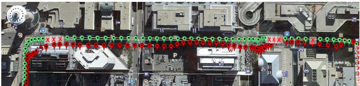
Figure 6-30: Last part of section three looking westward (Google, 2015)
