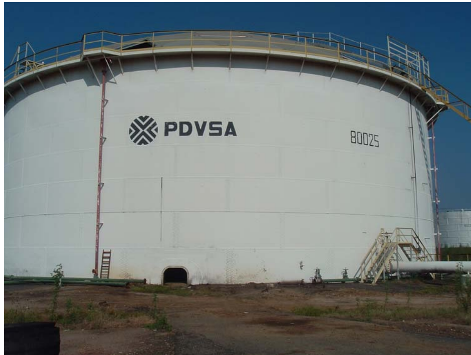
Figure 4.2 Typical oil tank in Venezuela
