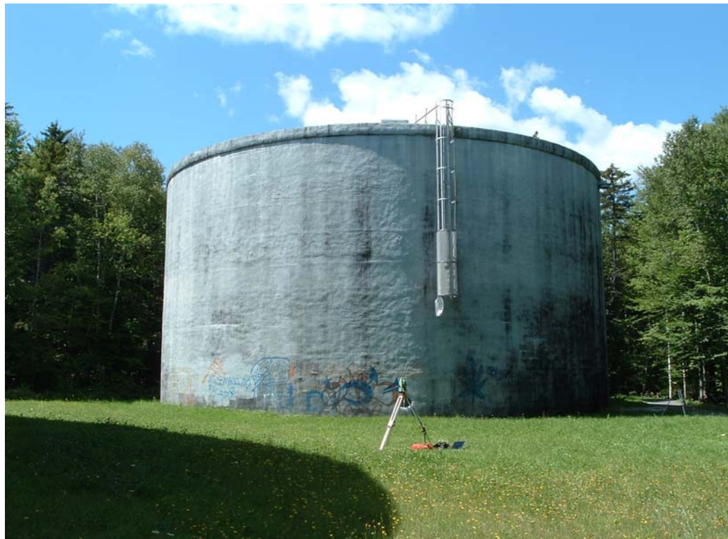
Figure 6.1 Water Tank in Fredericton, NB
