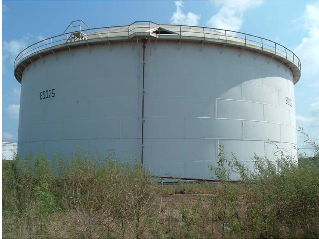
Figure 2.1 Typical large storage tank (approximately 15 m high)
