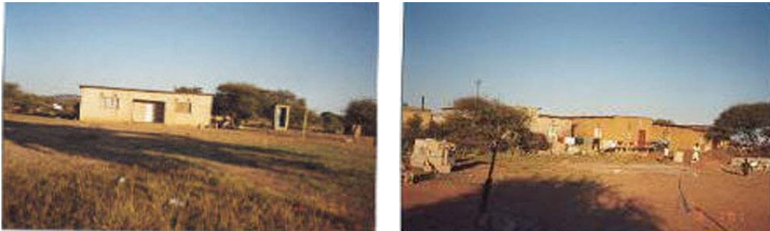
Figure II. 7: Examples houses marked for demolition usually painted with a red cross
