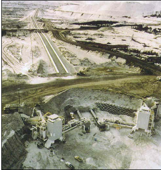
Figure 3.4 Crushers and Conveyor System [Mining Technology, 2003]
