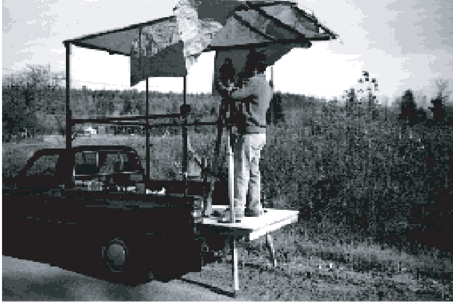
1985: Adam and his associates developed for the Geodetic Survey of Canada a motorized system for trigonometric height traversing of high precision. At the instrument (above) is Mr. A. Kharagani, a former UNB graduate student. The development included intensive studies on effects of tropospheric refraction. Below, Dr. A. Jarzymowski, a visiting scientist from Poland, and Mr. S. Vamosi, of the Geodetic Survey of Canada, are at an instrument for temperature gradient recording.
