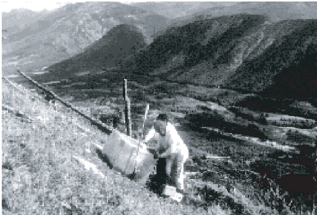
1980: Adam (right) and Dr. Yilmaz Fisekci of Canada Mineral and Energy Technology (CANMET) install a telemetric system for monitoring slope stability above an underground coal mine near Sparwood, B.C. This pioneering system, developed by Adam and his research associates for CANMET, allowed for a continuous monitoring of ground movements in the rugged terrain using an array of tiltmeters. The system was continuously operational for three years (1980-1983) at temperatures to -40^{\circ}\text{C} and under 3 m of snow during the winters.
