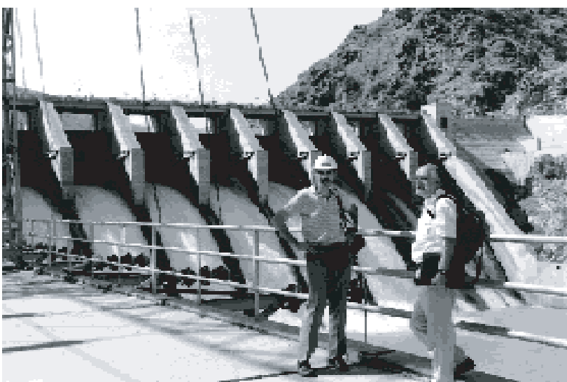
1996: Adam (right) at the Warsak hydro electric power station on the Kabul River in northern Pakistan. Adam and his graduate students designed and implemented an integrated survey scheme to monitor and analyse structural deformations and slope stability around the site. The project is to be completed in 2000.
