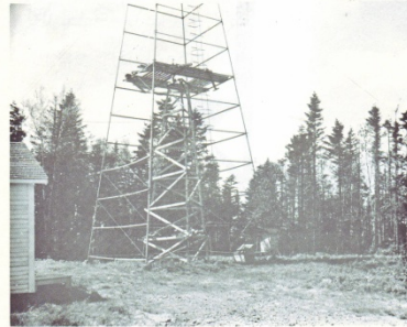
Wooden Instrument Tower of 30 ft. height Within Forest Service Steel Tower
